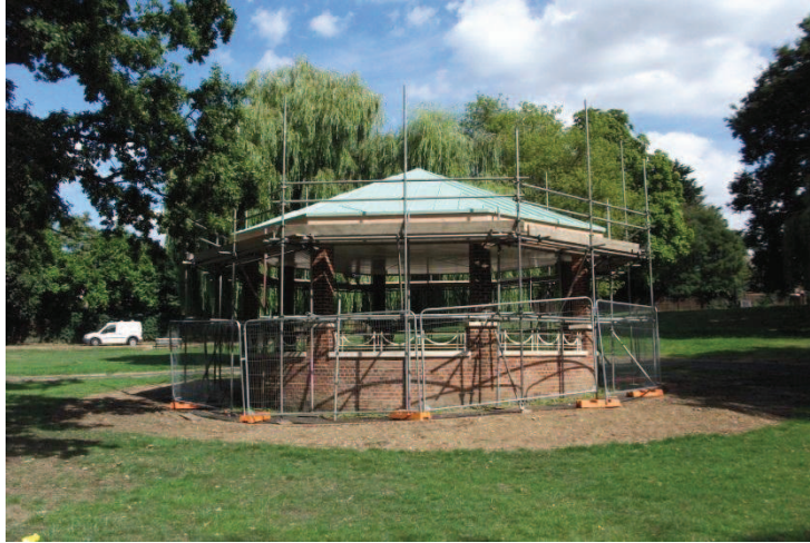
Bandstand Restoration Works in Raphael Park
